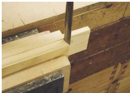
▲ Pic.17 The job is finished with a short scribing cut, which...
